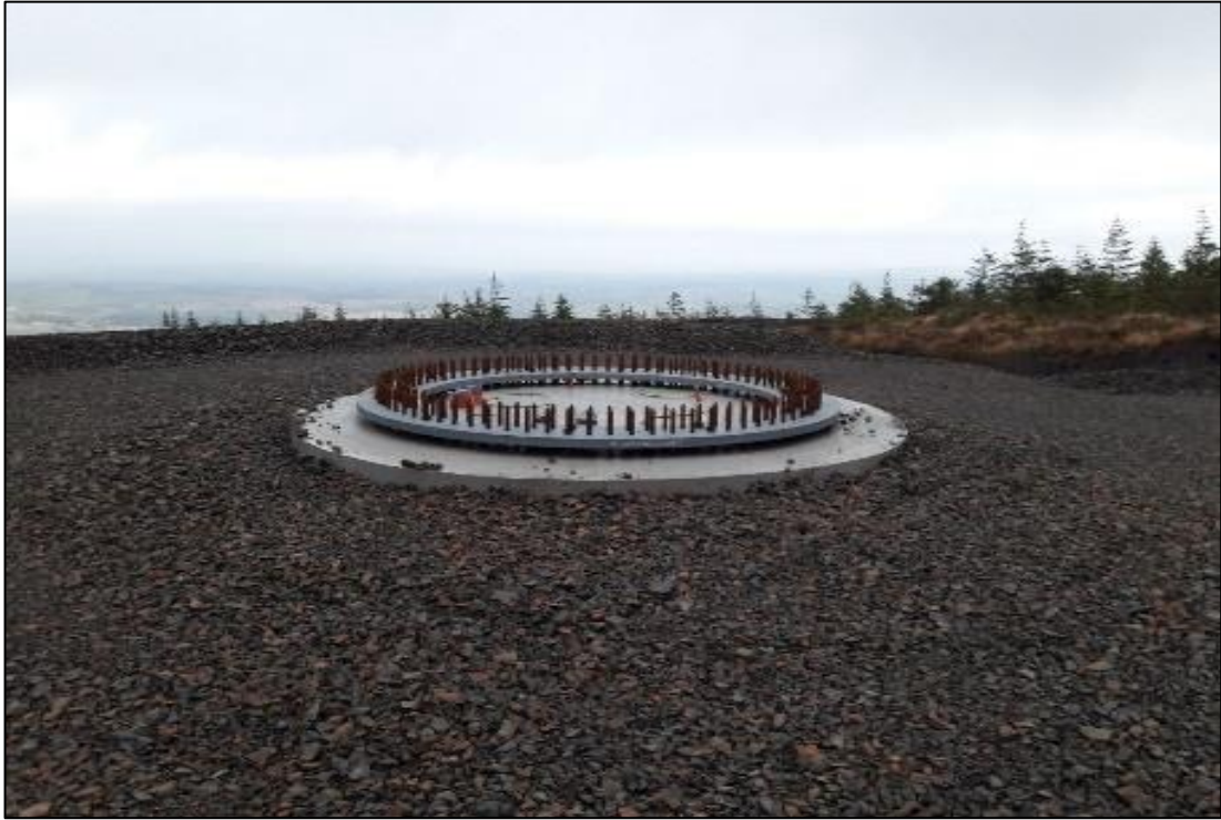
Plate 4-3 Finished Turbine Foundation
