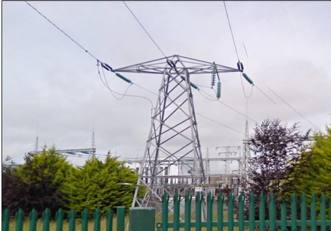
Plate 4-11 Completed End Mast Tower (example image)
