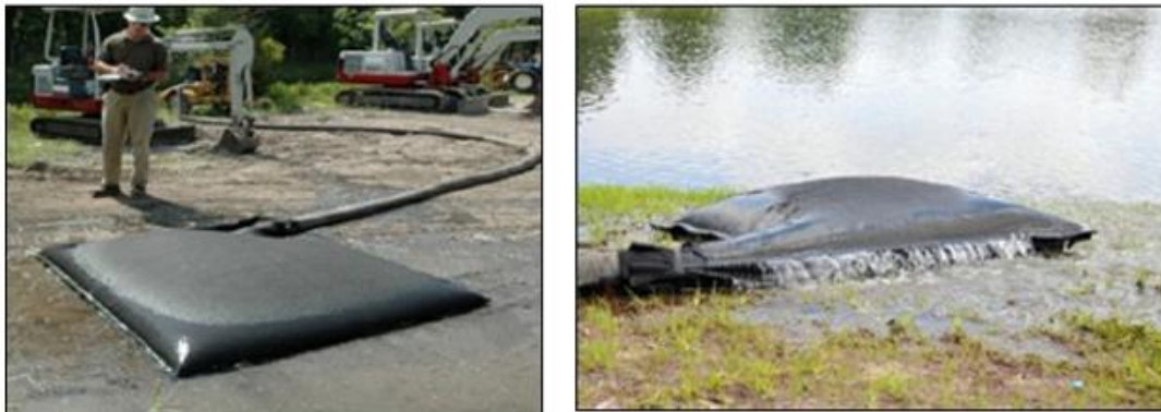
Plate 4-7 Silt Bag with water being pumped through.
