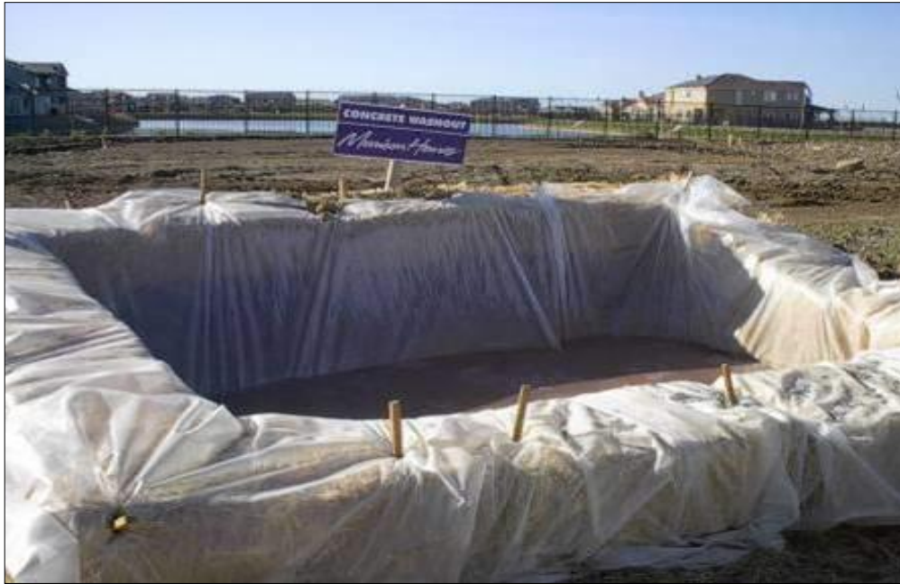
Plate 4-5 Concrete washout area
