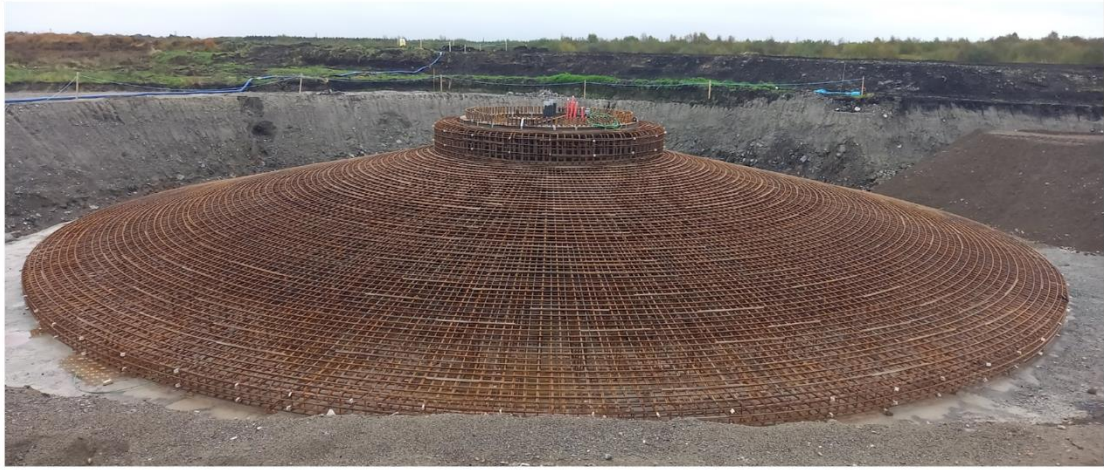
Plate 4-2 Turbine Foundation Anchor Cage surrounded by reinforcing steel.
