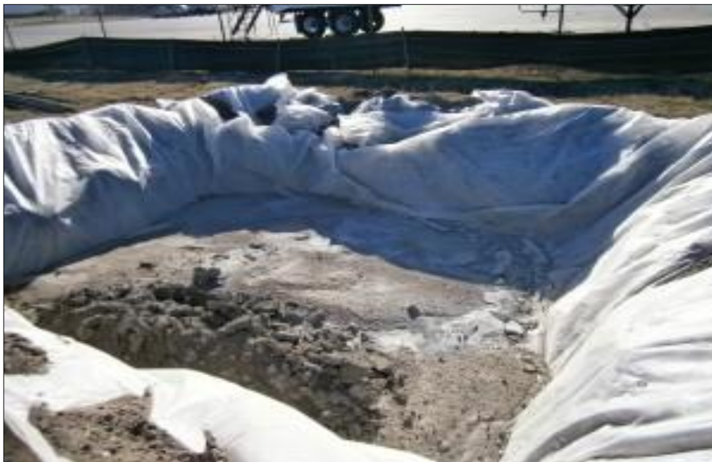
Plate 4-6 Concrete Wash Out Area
